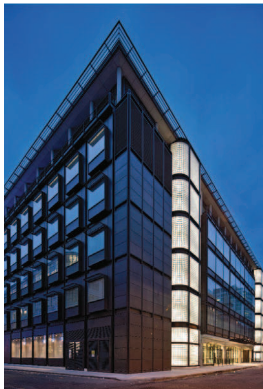
The Macmillan Cancer Centre at University College Hospital, which opened in April 2012.
